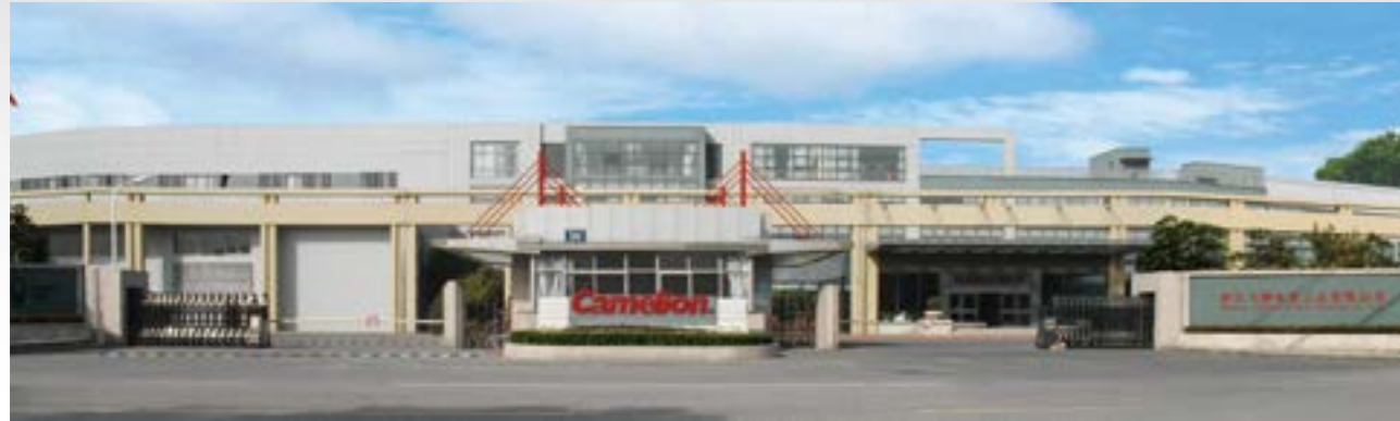
嘉兴碳碱性电池生产基地 Jiaxing Alkaline Battery Production Base
